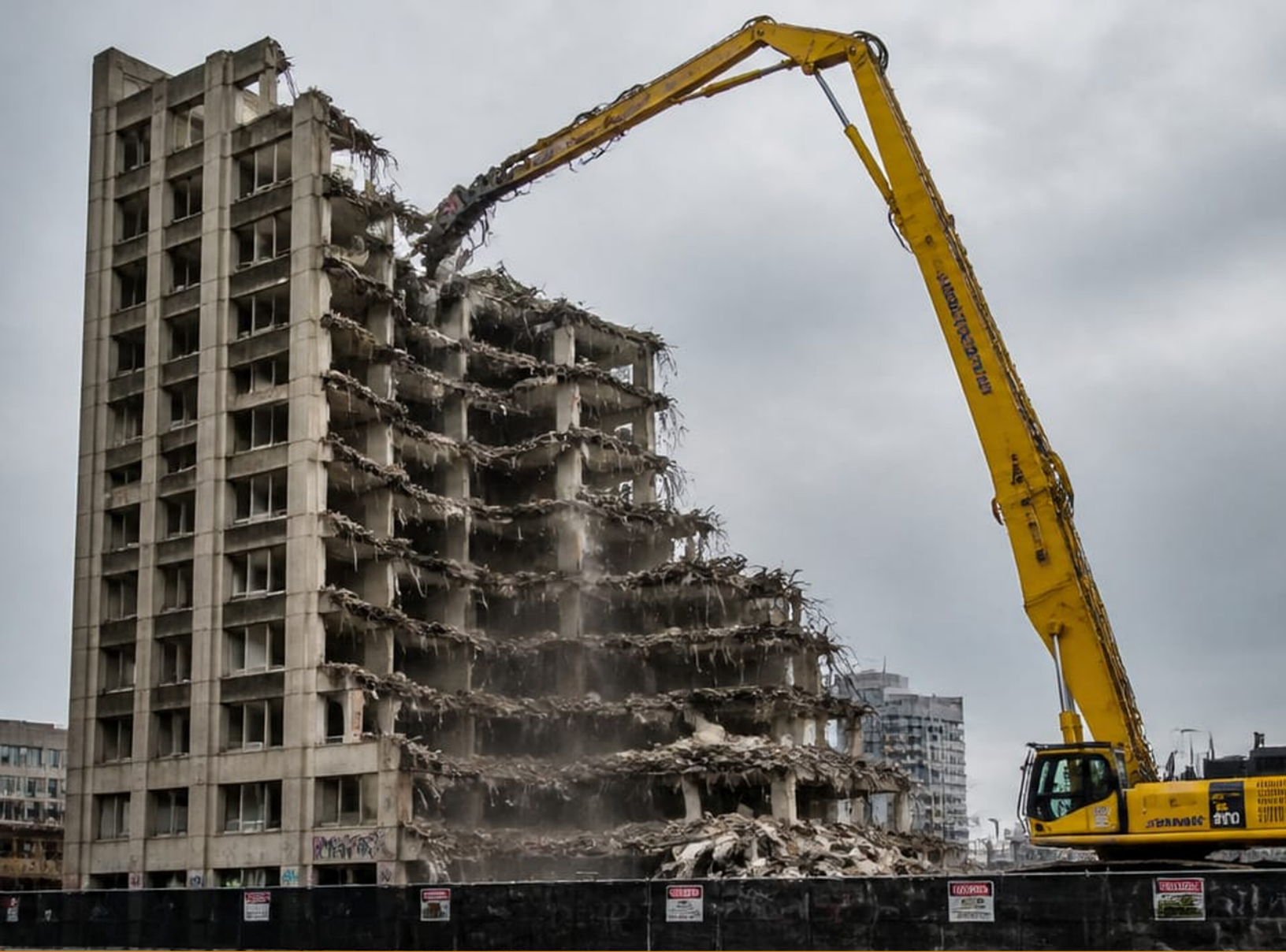
Komatsu PC800 Hydraulic excavator · 80-tonne operating weight
