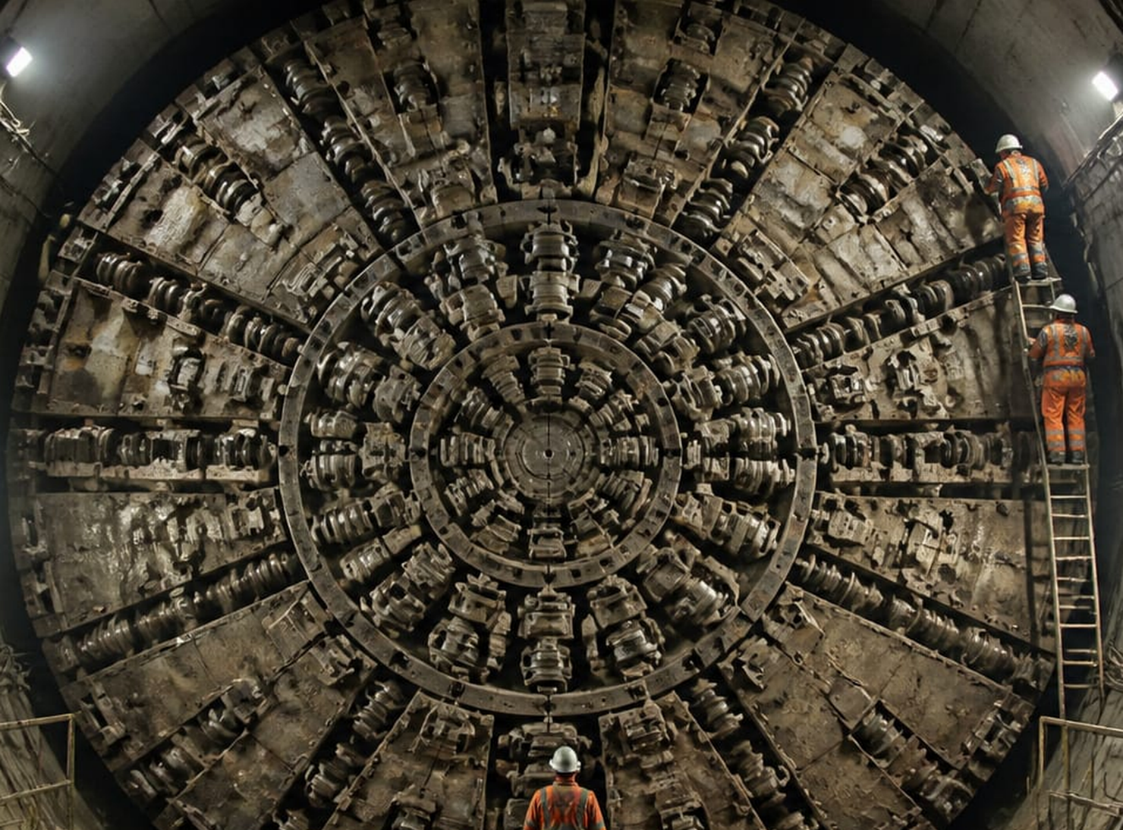
Tunnel Boring Machine Cuts through solid rock · diameter up to 19 metres
